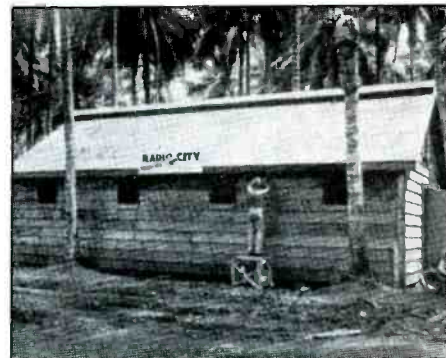
Stations in the "Mosquito Network" were often located at the sites of well-known WWII battles. This 20 by 40 ft. shed was the 1944 home of US Marine Corps station, "Radio Guadalcanal," in the Solomon Islands. The Program Director at the time was Spencer, W9GJL.
